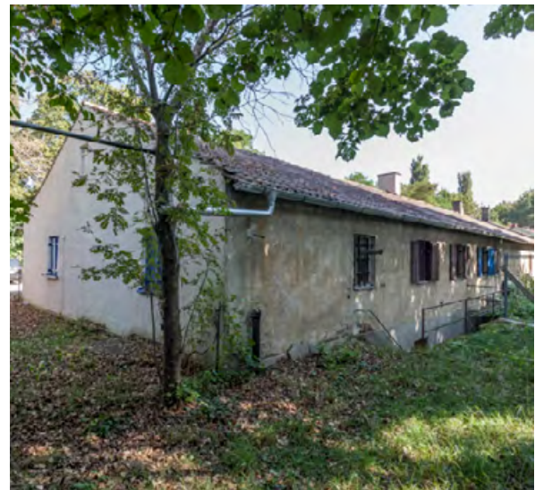
Another former barracks will house the branch of the Munich Documentation Center for the History of National Socialism
