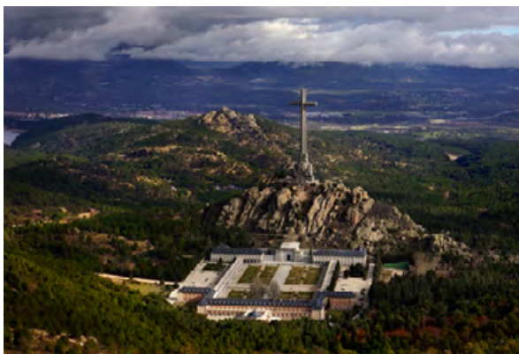
The building complex consists of a 152-metre-high concrete cross, a large parade ground, a Benedictine abbey, and a basilica
